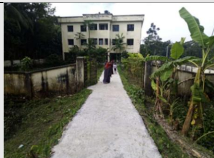
Photo: After construction the road of UHFWC
